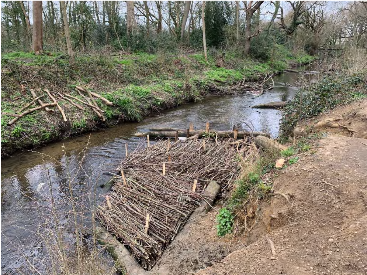
Creation of berms along a section the Beverley Brook located close to the 'Wooden Bridge'
